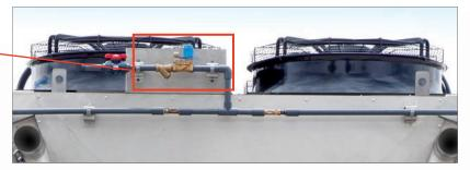
Adiabatic water supply solenoid valve arrangement
