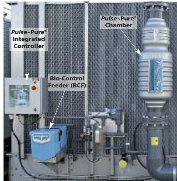
EVAPCO's **Pulse~Pure® PLUS** water treatment system utilizes pulsed electric field technology to provide an environmentally responsible alternative for the treatment of water in evaporative cooled equipment. The **Pulse~Pure® PLUS** system delivers short, high-frequency bursts of low energy electromagnetic fields to the recirculating water in the eco-ATWB-H.
