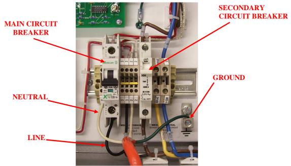
Figure 4 Supply power connections in 120V Pulse Panel with a circuit breaker
