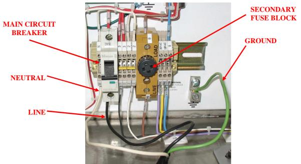
Figure 3 Supply power connections in 120V Pulse Panel with a fuse block
