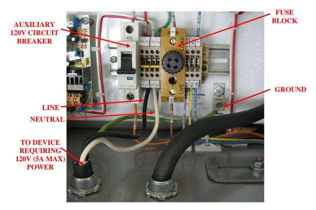
Figure 6 120V supply power connections in a 460V Pulse Panel
