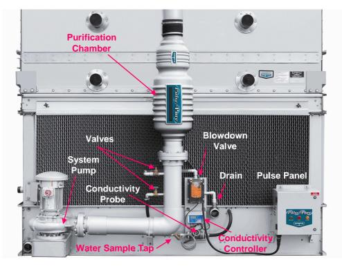
Figure 2 A typical factory installed *Pulse*~Pure<sup>™</sup> System with optional conductivity controller
