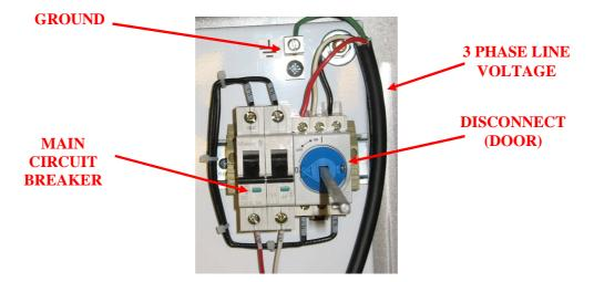
Figure 5 Supply power connections in a 460V Pulse Panel
