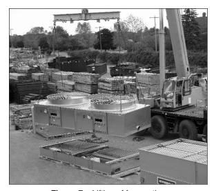
Figure 7 – Lifting of fan section
