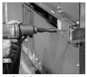
Figure 5 – Removal of shipping channels
