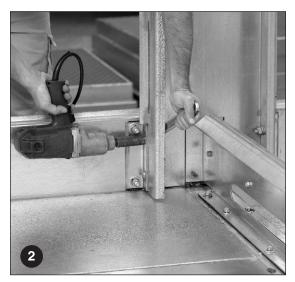
Step #2: Install vertical support and tighten hardware.
