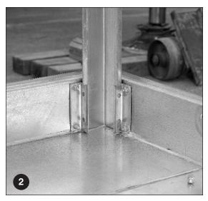
Step #2: Install corner vertical between brackets
