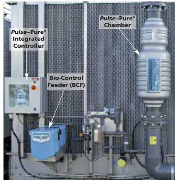
EVAPCO's **Pulse~Pure® Plus** water treatment system utilizes pulsed electric field technology to provide an environmentally responsible alternative for the treatment of water in evaporative cooled equipment. The **Pulse~Pure® Plus** system delivers short, high-frequency bursts of low energy electromagnetic fields to the recirculating water in the ESWB.
