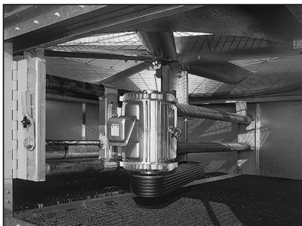
Motor Base Assembly
