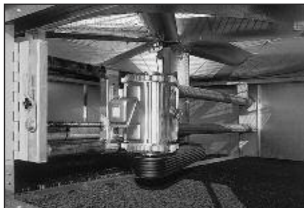
Motor Base Assembly
