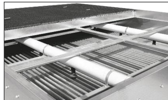
Drift Eliminators Removed for Coil Inspection
