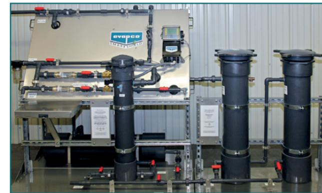
Fig. 4: Smart Shield® on Cooling Tower Application
