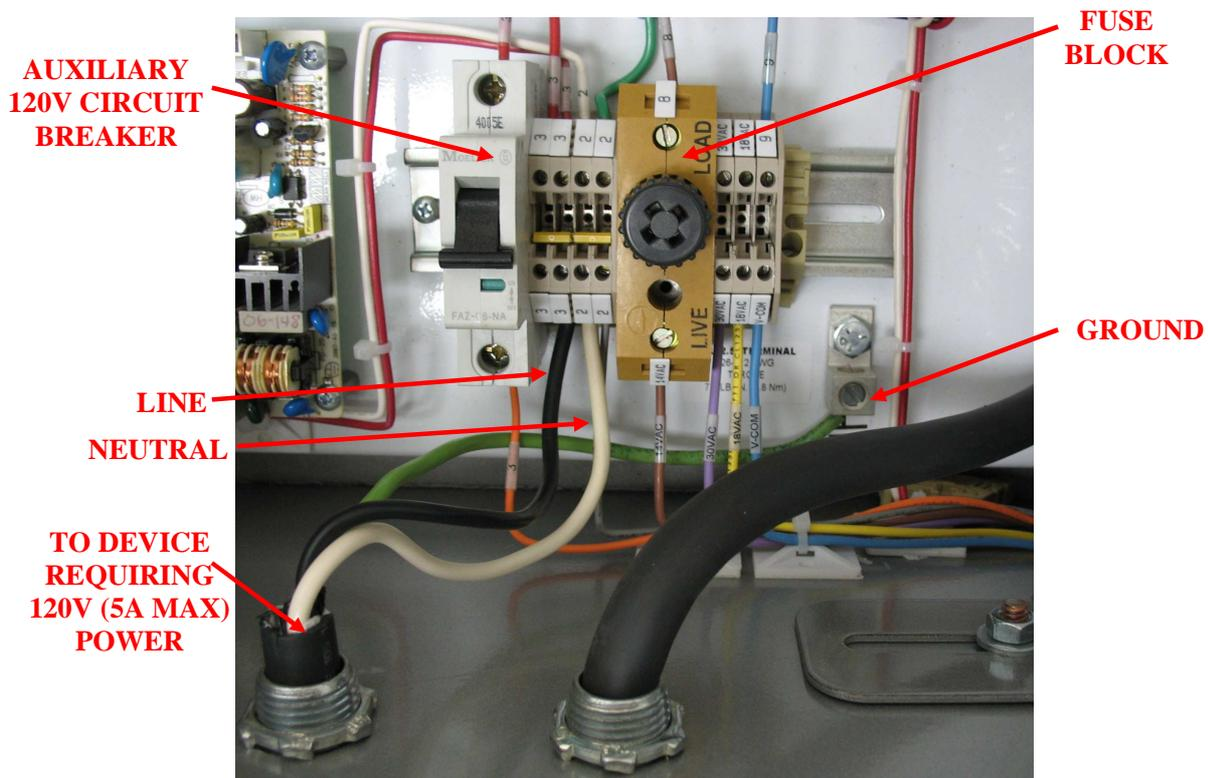
**Figure 6** 120V supply power connections in a 460V Pulse Panel
