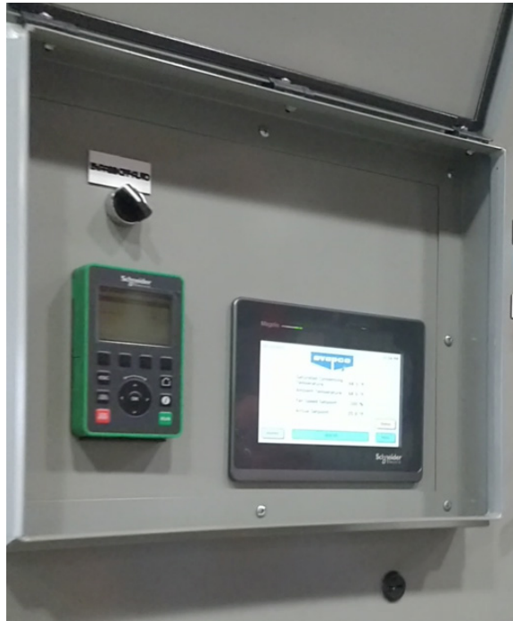
HMI, VFD and Bypass/ Off/Auto Switch for AC Motors
