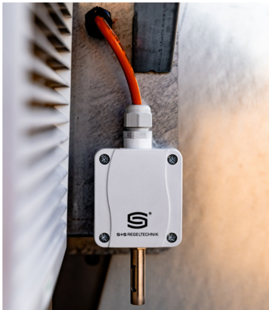
Temperature Sensor (Fluid Cooler)
