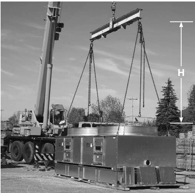
Figure 5 – Lifting arrangement for fan section
