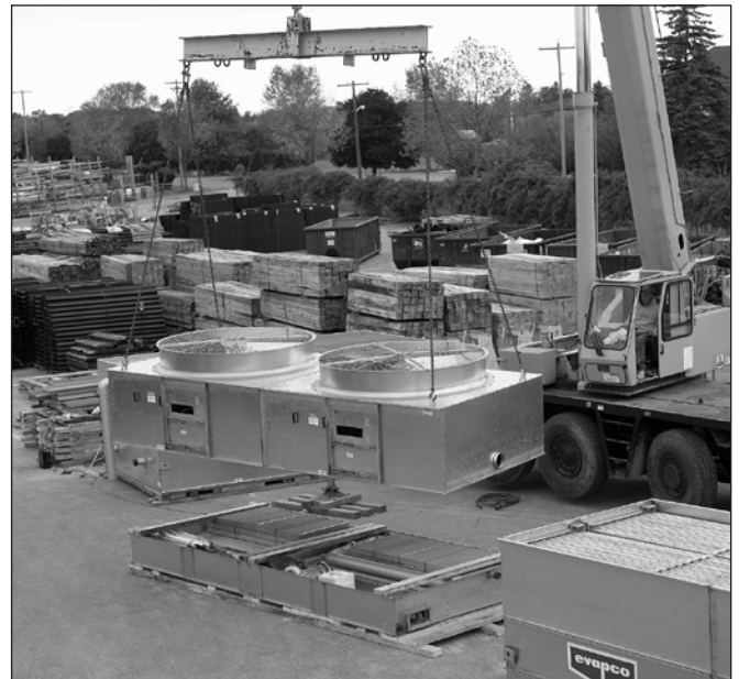
Figure 9 – Lifting of fan section
