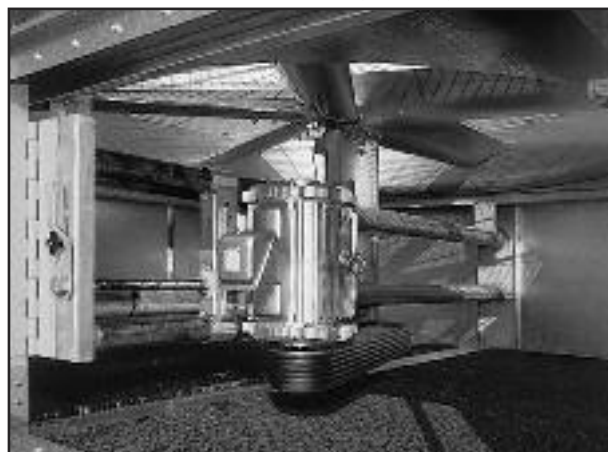
Motor Base Assembly
