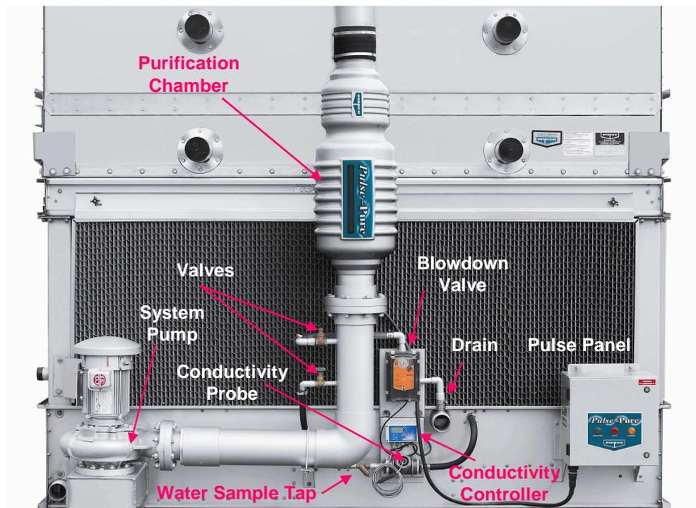
**Figure 2** A typical factory installed *Pulse~Pure™* System with optional conductivity controller
